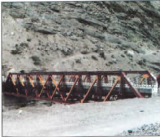
1. Attargu Bridge (A Gateway to PVNP)
